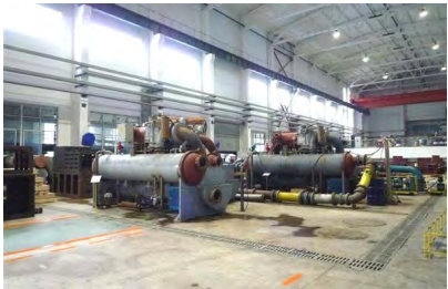
Commissioning of Centrifugal Chiller on site
