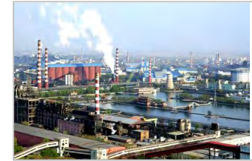
Capital Iron&Steel Group (2.4 million tons pellet project per year /fans)
