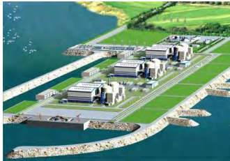
Fuqing Nuclear Power Station(Centrifugal Chiller)
