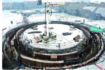
Wanjiashan Nuclear Power Station(Centrifugal Chiller)
