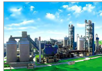
Gansu Qilianshan Cement Group (2500 tons of cement production line /fans)
