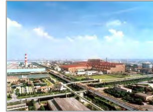
Shanghai Baoshan Iron&Steel Group (Silicon steel production line etc./fans)
