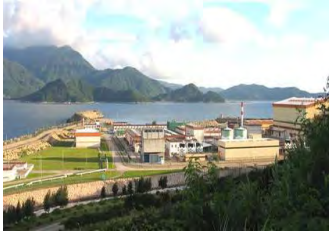
Daya Bay Nuclear Power Station (Centrifugal Chiller)
