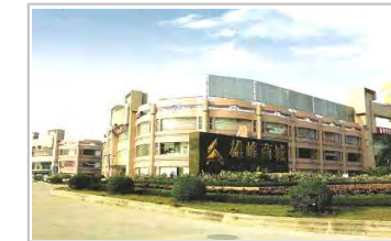
Guangdong Xiongfeng Mall (Centrifugal Chiller)
