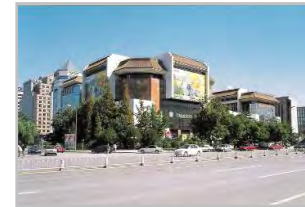
Beijing Parkson Mall (Centrifugal Chiller)
