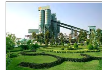
Guangxi Huarun Cement Group (2500 tons of cement production line /fans)
