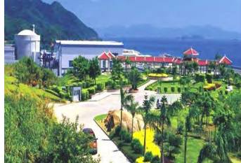
Lingao Nuclear Power Station(Centrifugal Chiller)
